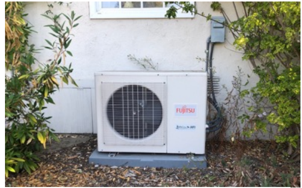
My heat pump model's outdoor unit can support up to two indoor units.
